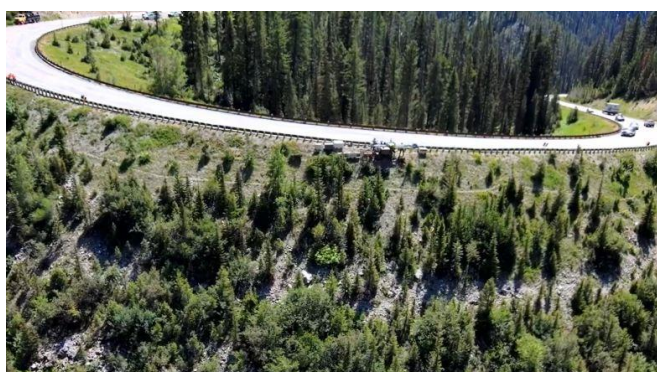
Screenshot from Wyoming Department of Transport footage of the site of the 6 to 8 June 2024 landslide on Teton Pass in Wyoming, USA.
