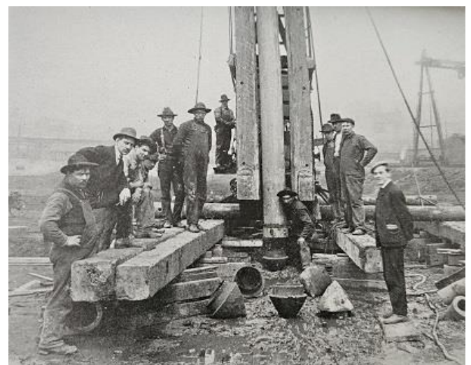
IMAGE 5: Simplex Concrete Piling Co. laborers pause for a photo while driving the firm's cast-in-place piles as shown in Image 4. Source: Simplex (1907).
