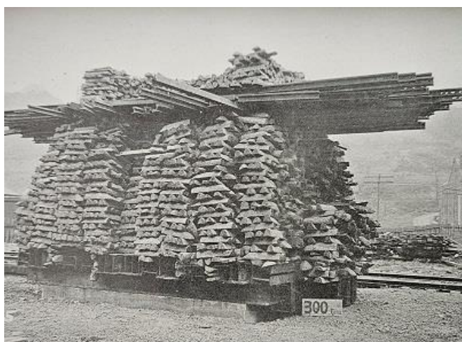
IMAGE 7: A static load test underway on a pile group for a crane at a Westinghouse plant, Pittsburgh, PA, 1905. Source: Simplex (1907).
