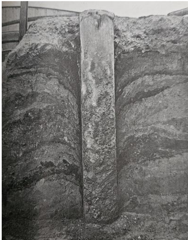
IMAGE 6: A cutaway of a pile and the surrounding soil after driving vividly illustrates the complexity of soil-static interaction during pile driving. Source: Simplex (1907).
