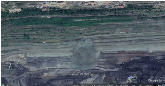
Google Earth image from May 2014 showing the failure at Fushun West OPM.
