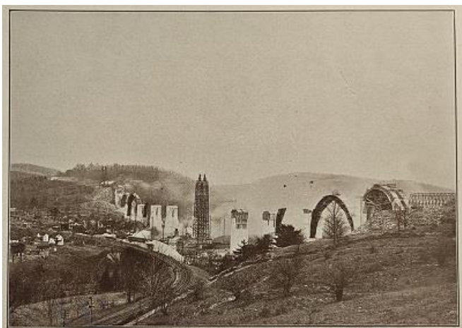
IMAGE 14: View of construction progress overall on the Tunkhannock Viaduct, fall 1913. Source: ASCE (1914).
