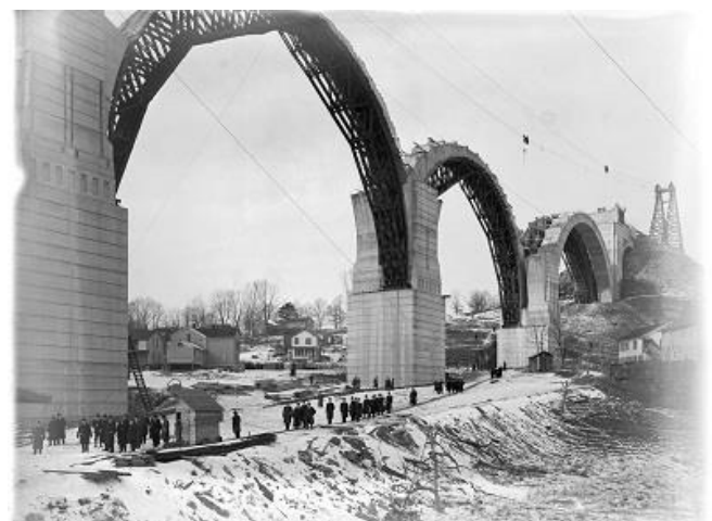
IMAGE 16: Civil engineers on the ASCE excursion train step out in derbies and fur coats to better view the construction of the Tunkhannock Viaduct. Source: NPS (2022).
