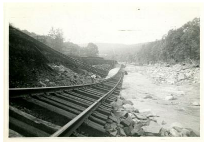
IMAGE 23: Damage to Lackawanna Railroad tracks in Scranton, PA, from Hurricane Diane, August 1955. Source: SPL (2024).
