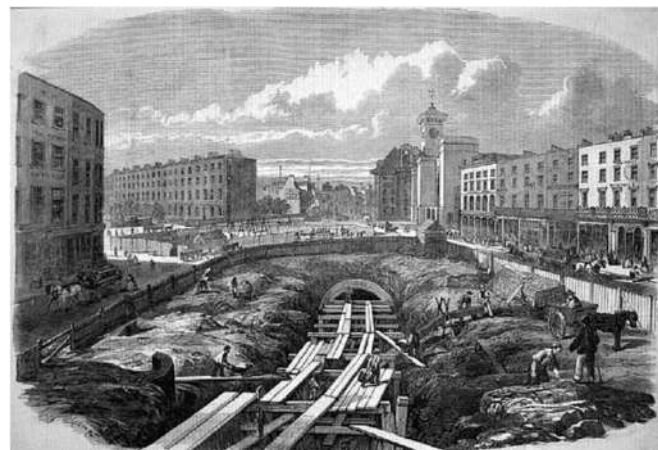
Painting by Percy William Justyn showing construction of the Metropolitan Railway, the world's first underground railway
