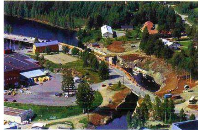
Fig.: 2: Juankoski: built lock and part of the channel
